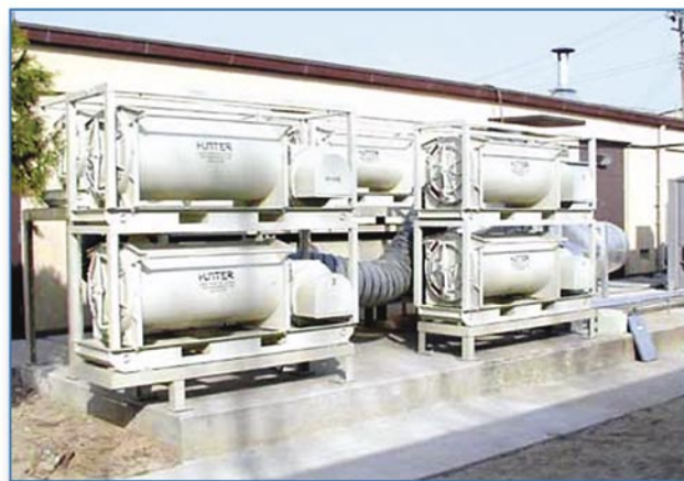
Figure 5-11 A military FFA 580 air filtration system containing both a HEPA filter and an ASZM-TEDA carbon adsorber as part of an overpressure system
